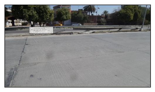
a) Transverse Tining PCC pavement surface texture (Section No.1)
